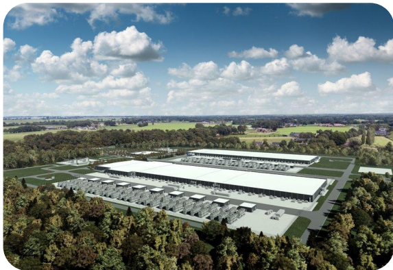
Project of META new AI datacenter in Temple, Texas (datacenterdynamics.com)
